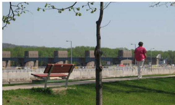
The walkway in Ingleside Park offers a place for pedestrians to walk as well as a scenic view of Lock and Dam No. 10.
